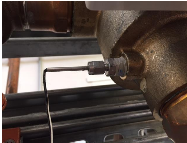
INSTALLATION OF COMPRESSION FITTING AND OUTLET RTD PROBE ON 2" NUCLEUS VALVE BODY
